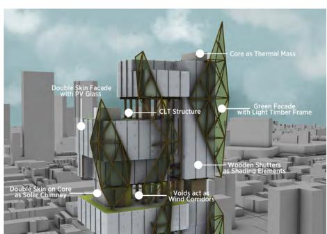
PV Panels are put on the surface of the solar chimney, and some of the glasses on the East-West facade are PV glass.
