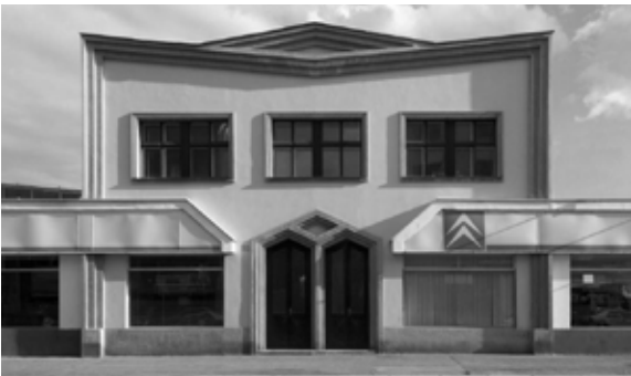
Rudolf Stockar: Materna Factory and Administration Building in Prague 7 / 1919-1920
