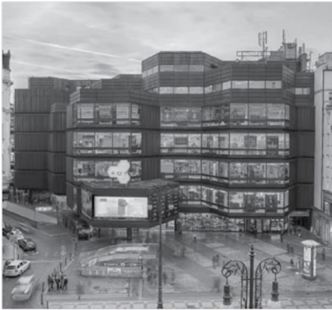
Kotva Department Store, Prague, 1975
