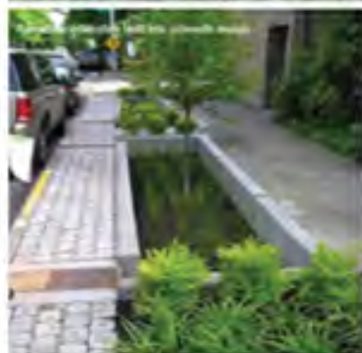
Rainwater infiltration system that emits water by the help of the plants.
