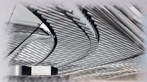
Construction of Space
