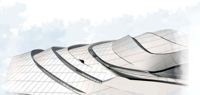
Roof is tilted to south to catch natural light & summer breeze & closed at north side to block north winds
